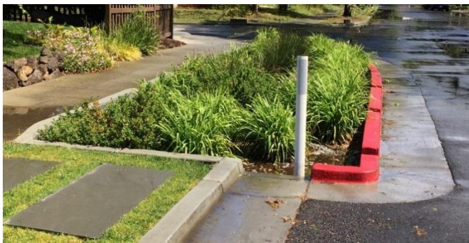
UNLINED BIORETENTION AREA WITH UNDERDRAIN, SOUTHGATE NEIGHBORHOOD STORM DRAIN IMPROVEMENT AND GREEN STREET PROJECT, PALO ALTO, CA (SOURCE: EOA, INC.)
