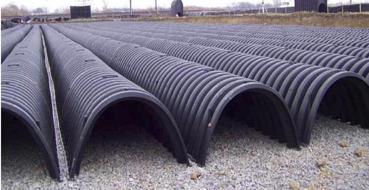
SUBSURFACE INFILTRATION SYSTEM INSTALLATION UNDER A PARKING LOT (SOURCE: CONTECH)
