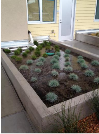
FLOW-THROUGH PLANTER (SOURCE: EOA, INC)
