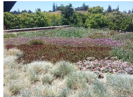
GREEN ROOF, DAVID AND LUCILLE PACKARD FOUNDATION HEADQUARTERS (SOURCE: CITY OF LOS ALTOS)
